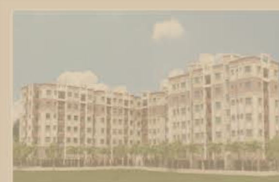
GREEN OASIS - KAIKHALI, KOLKATA
